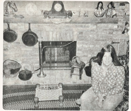
Gail Van Vark Kirby in the Tuttle Cabin. The brick fireplace replaced the original coal stove.
