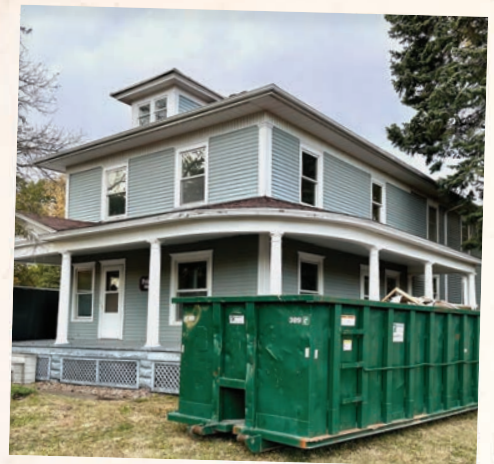
Renovation work by the Dykstras is underway at the Prins House.
