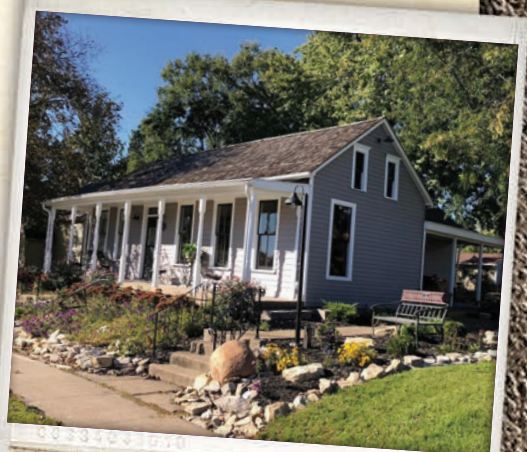
Saved from the bulldozer with funding assistance from philanthropist Joan Kuyper, this prototypical early Pella home was stabilized by the Trust and sold with a conservation easement.
