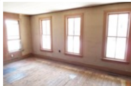
Removal of panelling revealed wide window trim.
