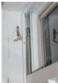
Parting stop and completed window.
